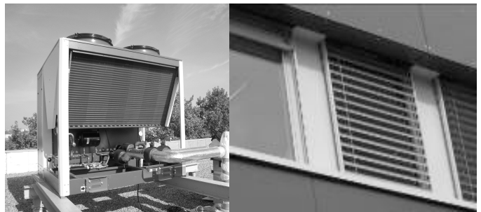
Figure 2: Details of the renovation: heat pump and solar shading device
